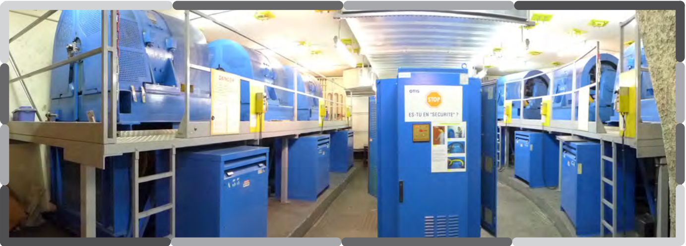
Upper bank machine room before
