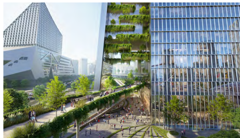
The gap between the leaning volumes leaves room for balconies and ground-floor public spaces; image courtesy of BIG.
