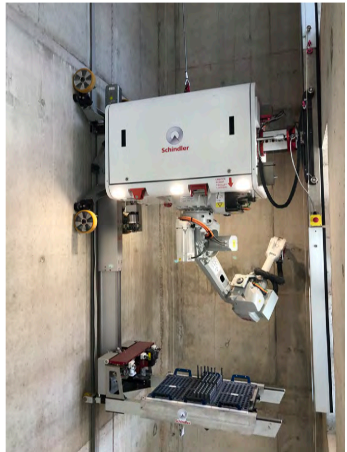
Installation robot Schindler R.I.S.E at work; courtesy of Schindler
