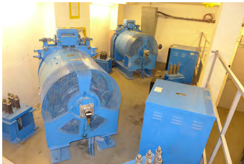
Lower bank machine room before
