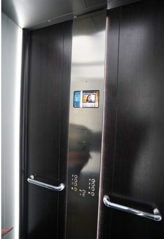
Latest eVIEW emergency call technology in a Gen2 cabin on the way to Udo Hoffmann; source: Hans-Wilhelm Berghoff
